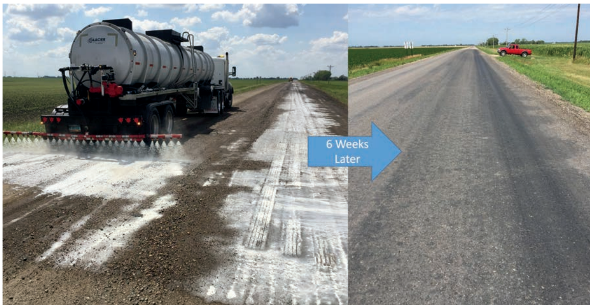
Soy-based road dust control applied to a gravel road containing RAP (left), The same gravel road 6 weeks later transformed into an “asphalt-like” surface (right).
