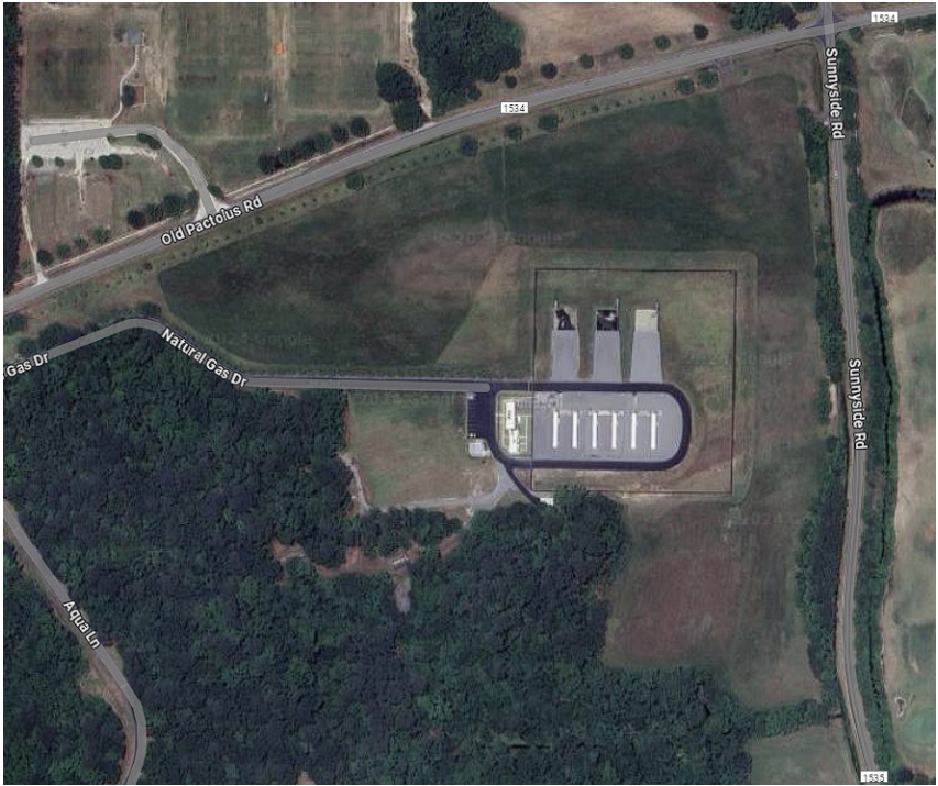
FIGURE 1.24 GREENVILLE MUNICIPAL UTILITIES ABOVEGROUND STORAGE TANKS 220
