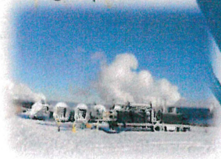
Interim LNG Storage at Wahpeton Injection Point
