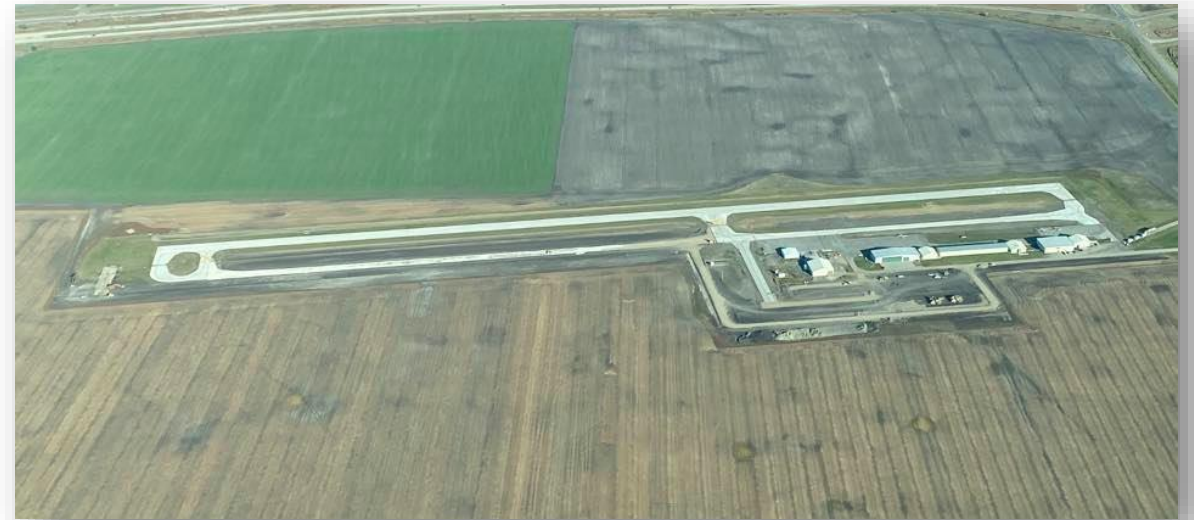
Hillsboro taxiway construction (2020)
