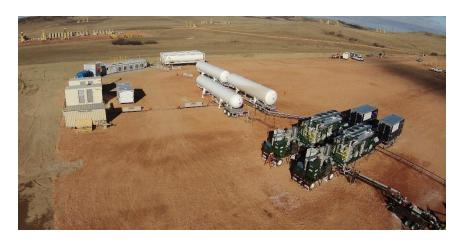
Figure 5: 2 MMCFD of installed GTUIT flare capture equipment along with well site LNG production
