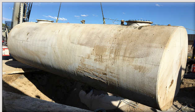
Removing an underground storage tank
